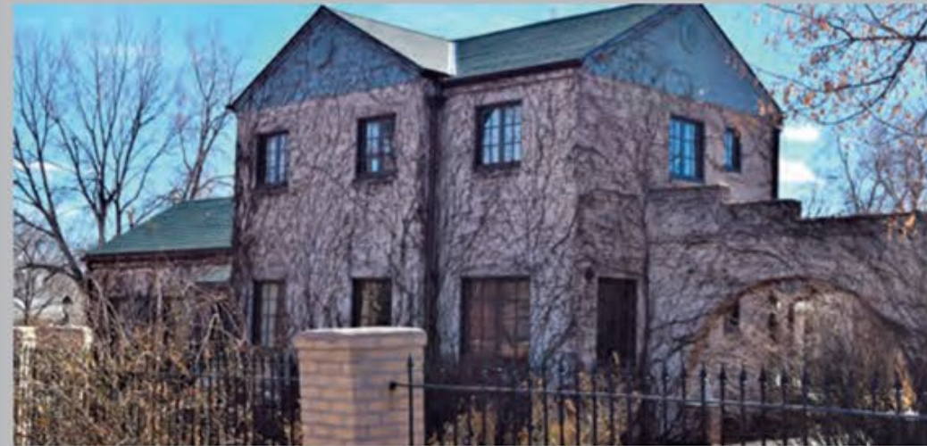
Sub-style of Tudor Revival. Usually two stories with only a single exterior material. Quite rare in Colorado. Common elements: steeply pitched roof, intersecting gables or dormers, front facade chimney, arched entrance, casement windows with heavy mullions, half-timbering, decorative brickwork, diagonally set chimney stacks. (Image: 9200 Lombardy Ln.)
