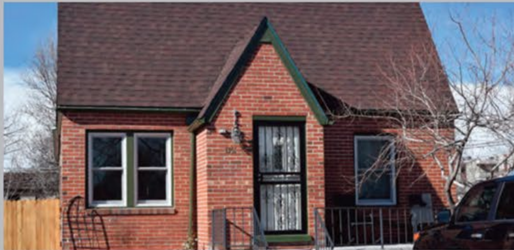
Modest, simplified version of the Tudor Revival style. Often built as an alternative to the Bungalow. Common elements: steeply pitched roof, steeply pitched gable entrance, decorative brickwork, arched entrance, stucco or brick exterior, casement windows, large front picture window, multi-light windows. (Image: 1351 Brentwood St.)
