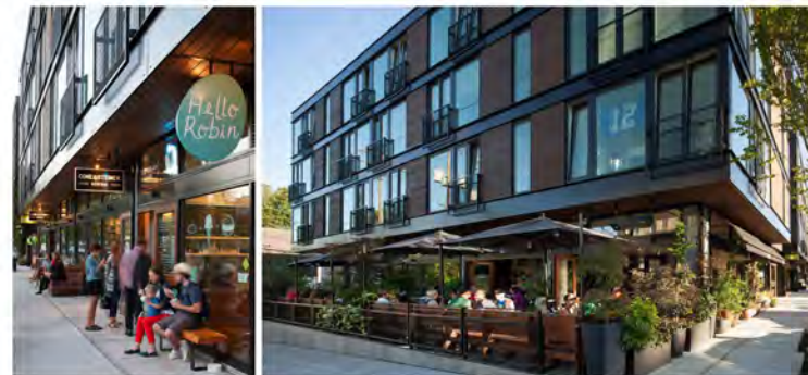
Examples of Ground Floor Building Design and Building Materials and Articulation to be included in the Design Standards & Guidelines
